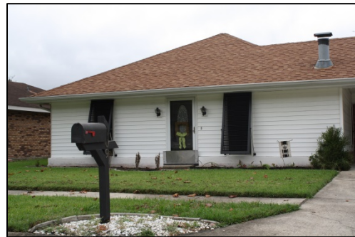
Figure 26 - This Bayou Cane home has a steel door to keep flood waters out.
