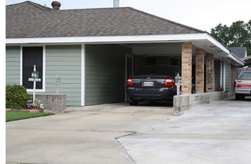
Figure 21 - This home is surrounded by a floodwall that doubles as a planter. The driveway must be sandbagged during a flood event.
