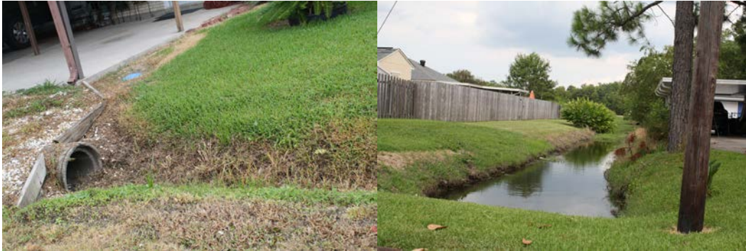
Figure 7 - Examples of Culverts and Ditches found in Bayou Cane
