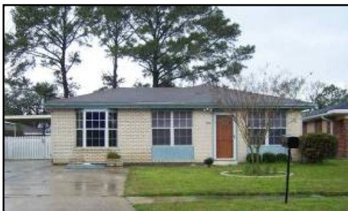
Figure 27 - This dry floodproofed building in Mandeville, LA has the walls waterproofed and removable shields placed in the windows
