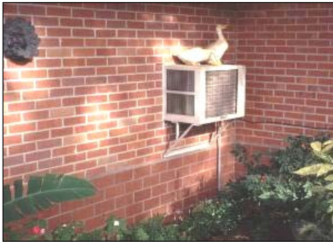
Figure 25 - This Baton Rouge, LA home had thin facing brick placed over the waterproofing materials.
